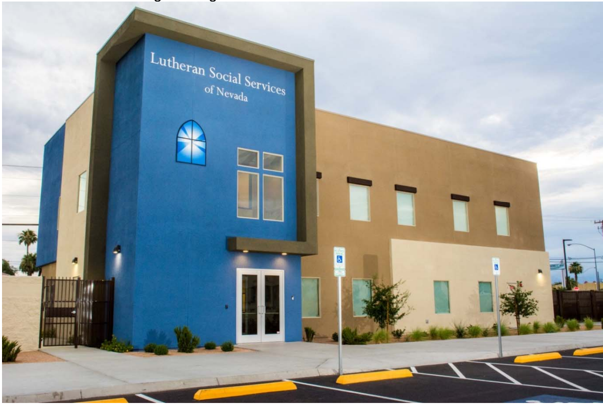
The existing building for Lutheran Social Services of Nevada
